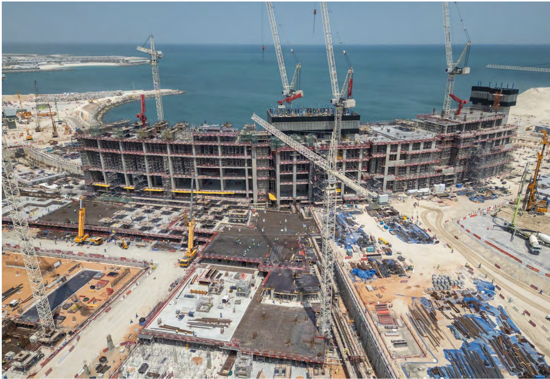
Construction Progress as of April 2024
